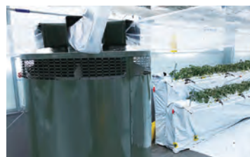
Heat exchanger for warming greenhouses and plant roots
