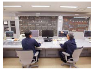
Central monitoring system at the Central Energy Plant
