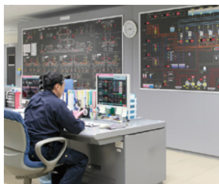
The central monitoring system for our central energy plant
