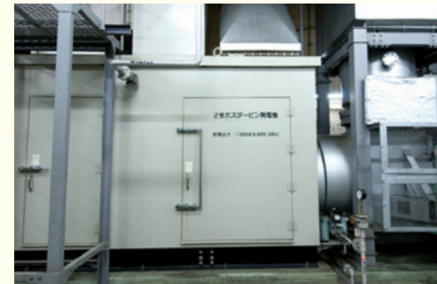
Power generators run on natural gas
