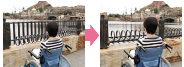
Movable safety fence that does not obstruct the view of Guests using wheelchairs
