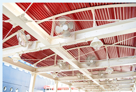
Misting fans and electric fans installed to alleviate the heat based on Guest feedback
