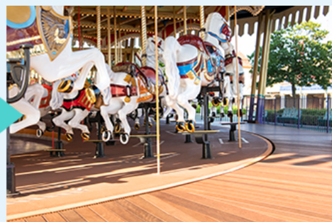
The floor surrounding the turntable was raised to eliminate height difference.
