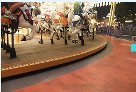
The floor surrounding the turntable was raised to eliminate height difference.
