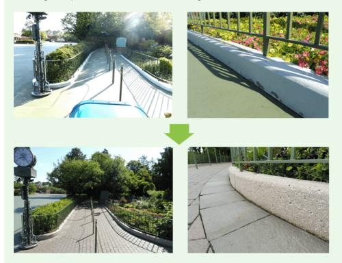
Applied no paint to the curbstone and eliminated chemical substances from pavement materials
